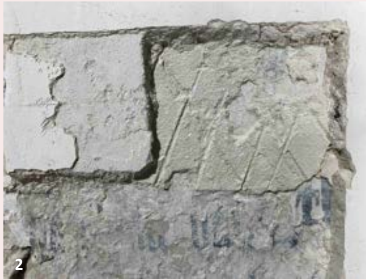
Left: Stages in uncovering of the painting from beneath the C19 plaster: (1) initial chiseling of overlying plaster, revealing its application in two layers, the lower one scored to receive the upper layer; (2) gradual uncovering and thinning of overlying materials, layer by layer; (3) thinning of remaining covering material; and (4) after uncovering.
