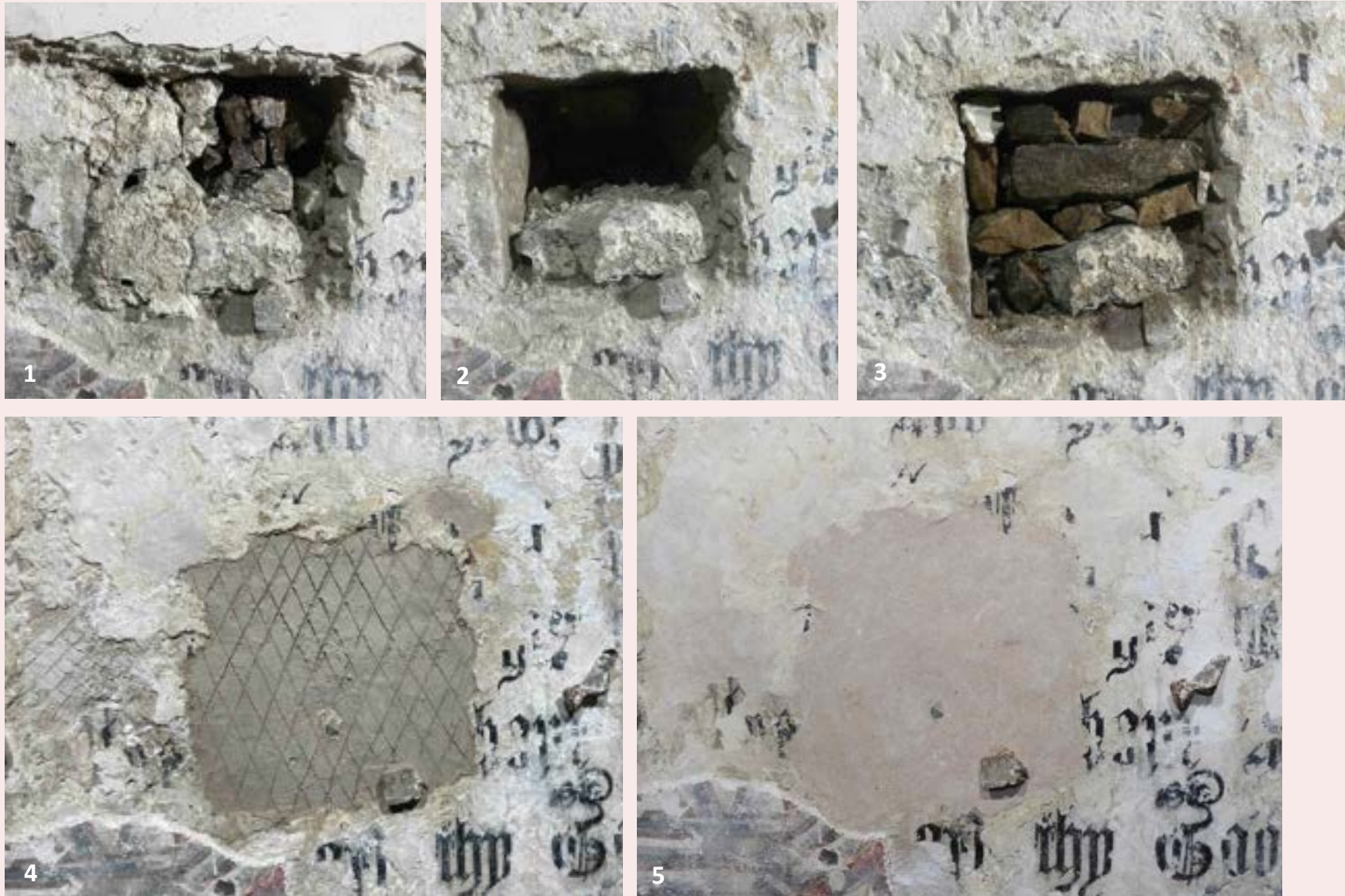
Above: Stages in making repairs: (1) put-log hole randomly filled with stone pieces and wood, as found after uncovering; (2) during removal of loose filling materials; (3) reinsertion and packing of filling materials and pre-wetting; (4) after application of lower coarse plaster; and (5) after application of upper fine plaster.
