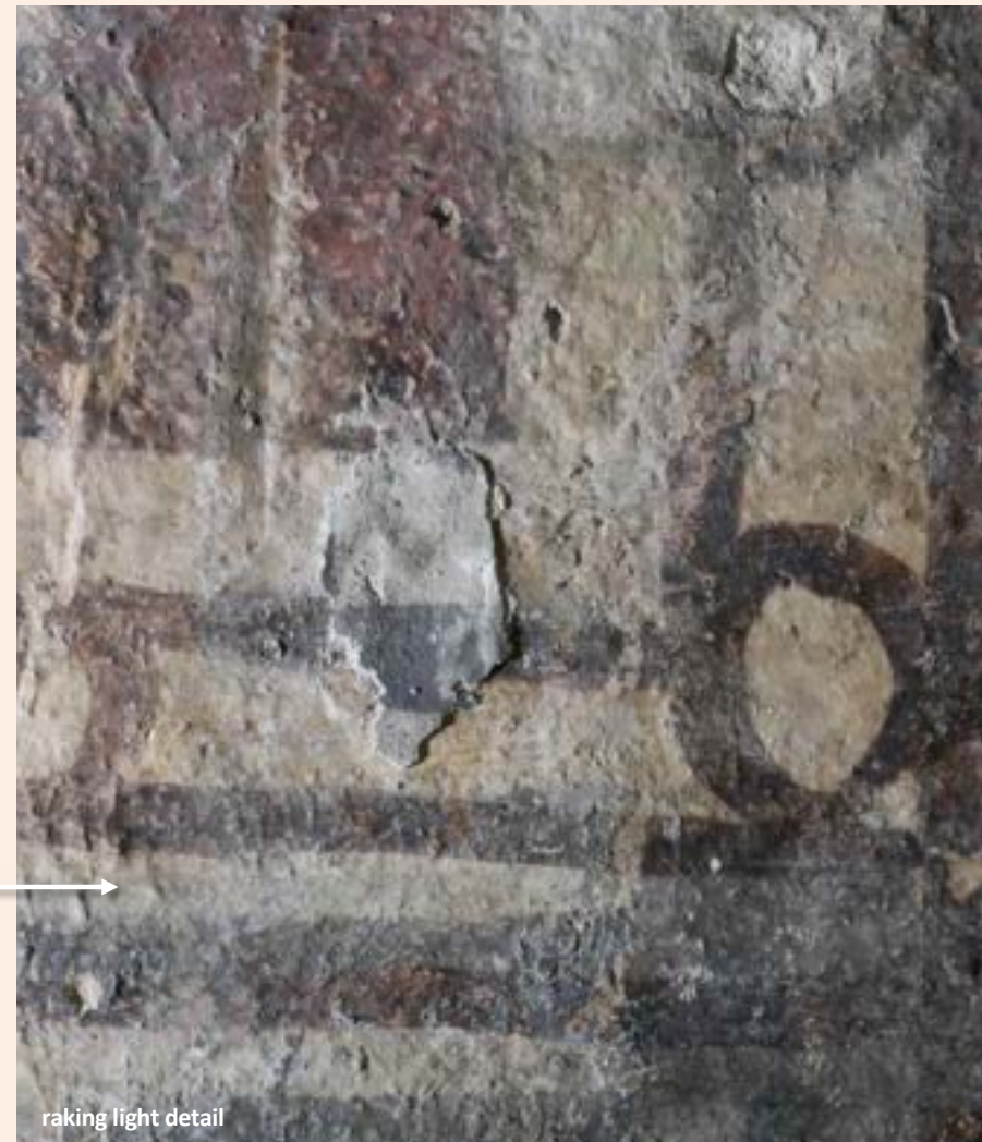
Left and Above: Very small traces of what appears to be a black-letter text painting survive on a limewash layer on top of the architectural fragment.
